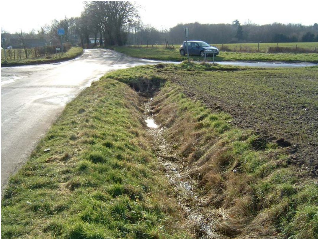
Figure B.15: Crown Road Drain, looking downstream and junction with Ragmore Road
