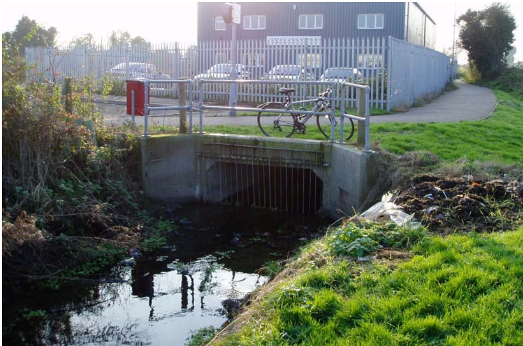
Figure A.7: Entrance to Maurice Gaymer Rd Culvert
