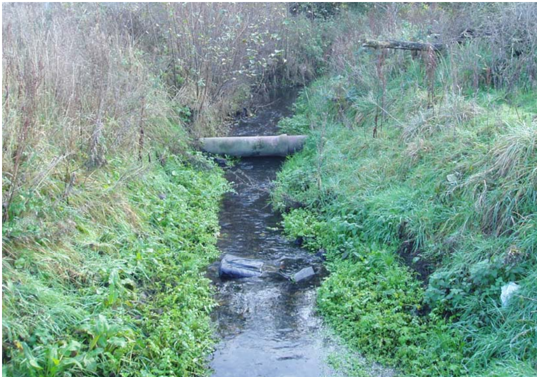
Figure A.9: Looking downstream from Maurice Gaymer Rd Culvert
