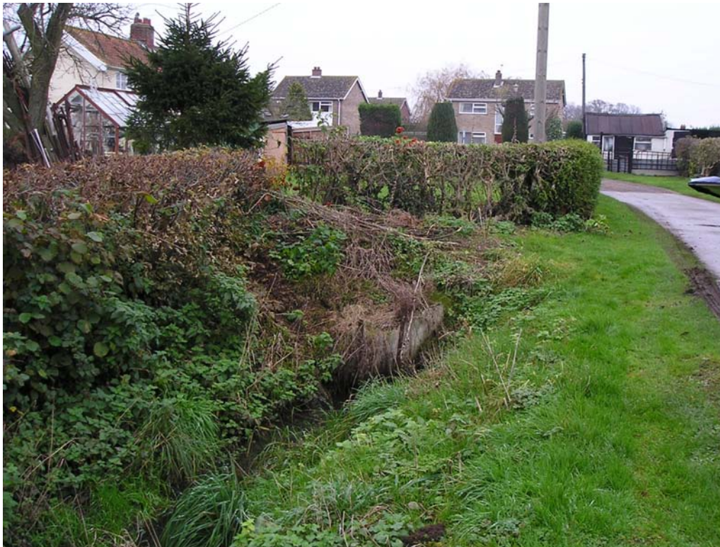
Figure B.17: Watery Lane Drain looking Downstream
