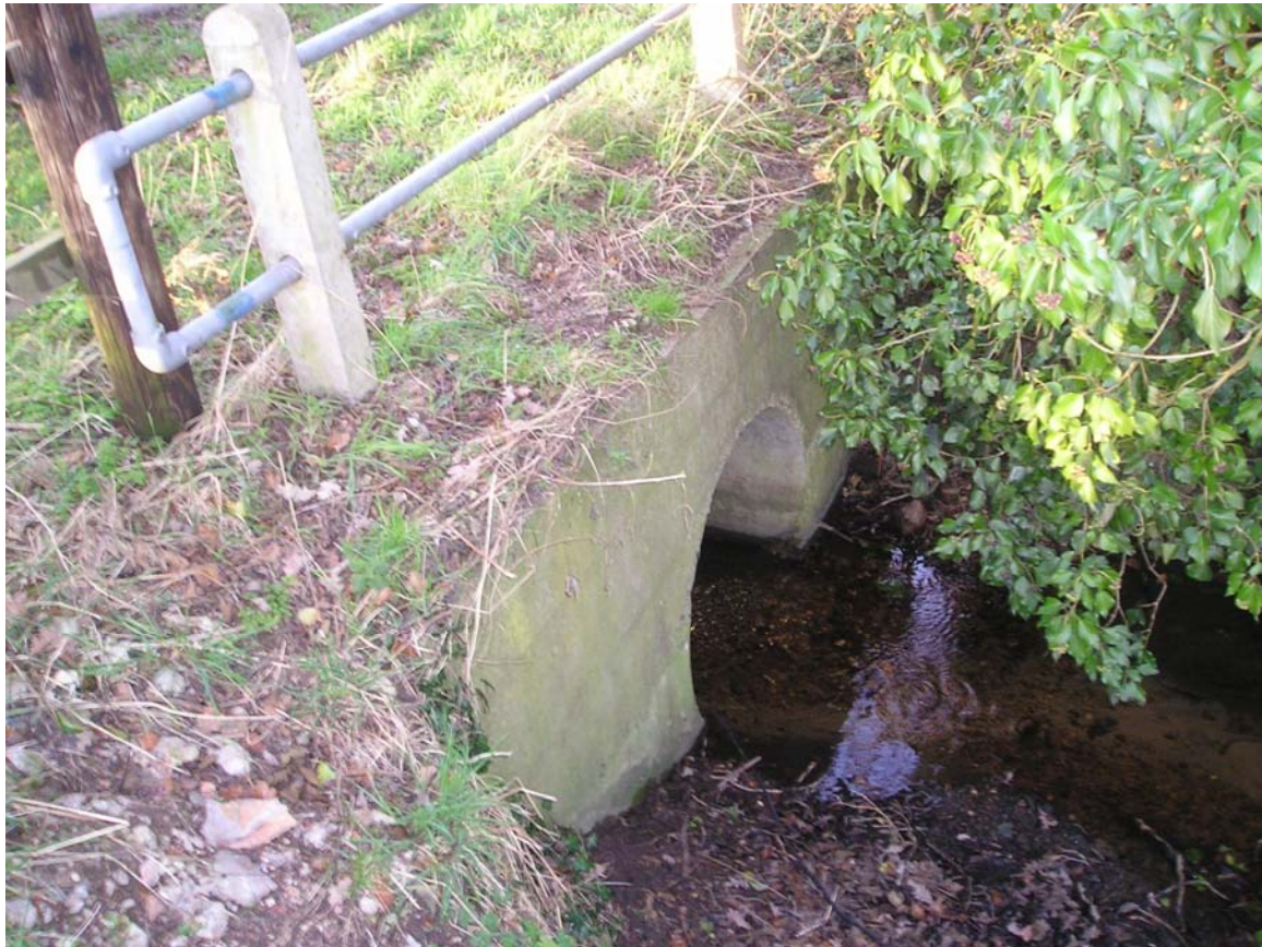
Figure B.4: Mauley's Drain showing upstream end of Culvert under West Harling Road
