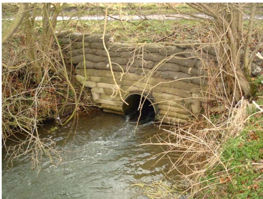
Figure B.12: Culvert under Farm Track
