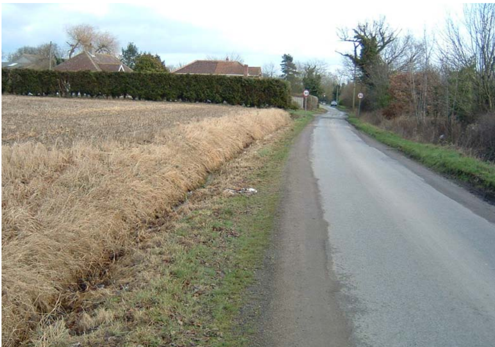
Figure B.3: Penhill Lane Drain adjacent to the road looking downhill
