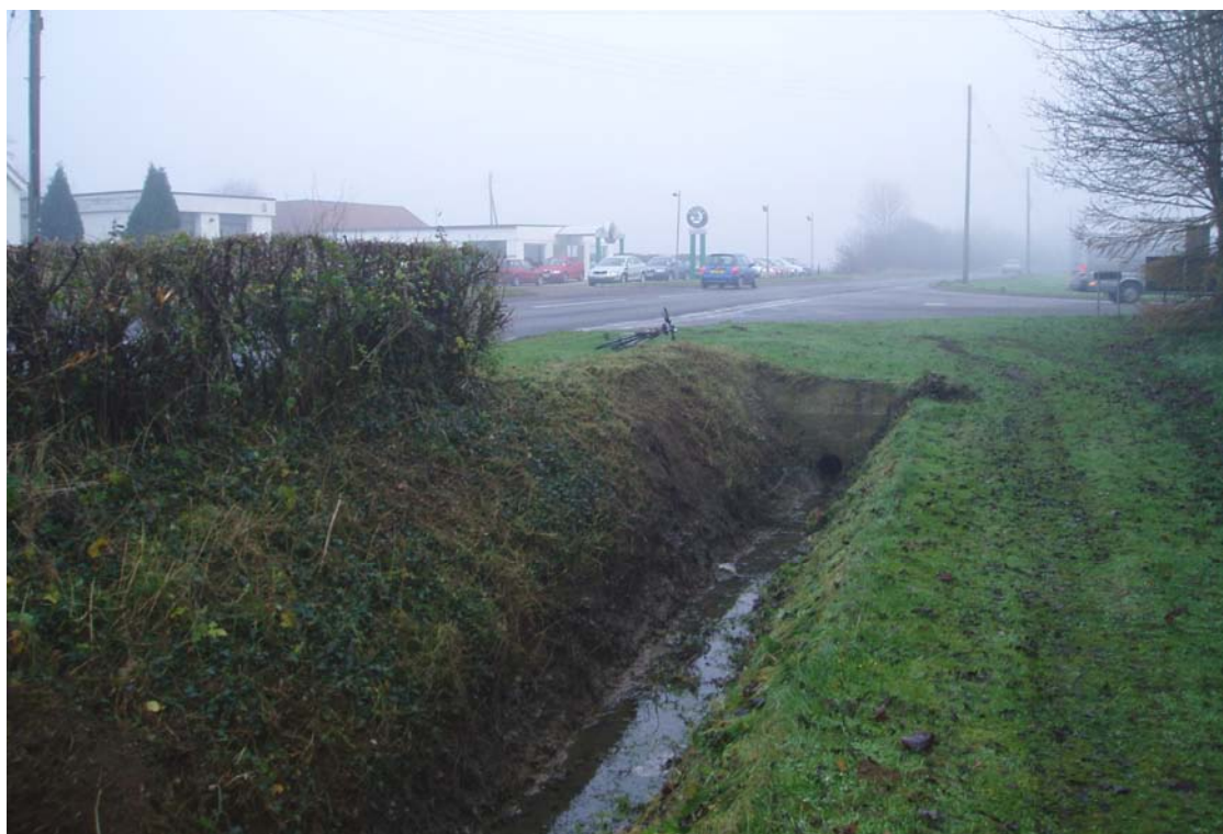
Figure A.13: London Road Ditch adjacent to Haverscroft Industrial Estate
