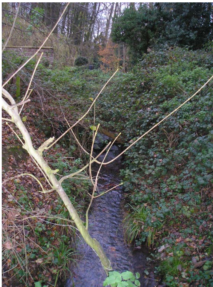
Figure B.18: Parkland Stream behind Parkland Avenue, looking upstream
