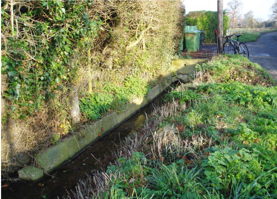
Figure A.3: Whitehouse Lane Drain looking upstream (east) adjacent to property
