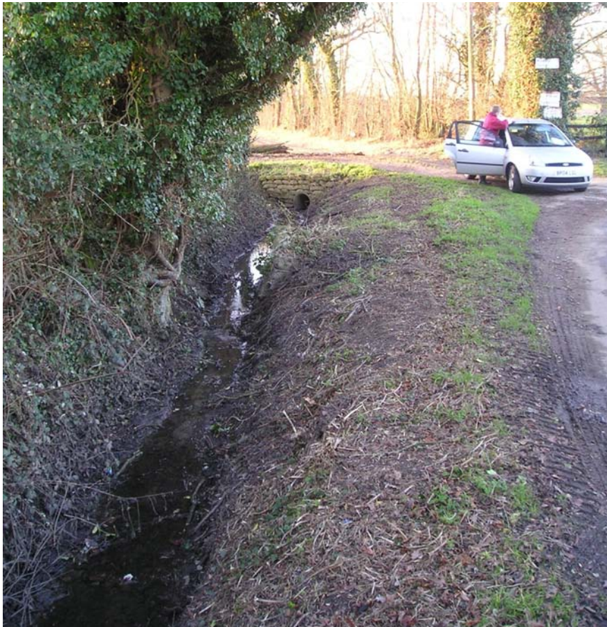
Figure B.6: Occupation Road Drain looking downstream
