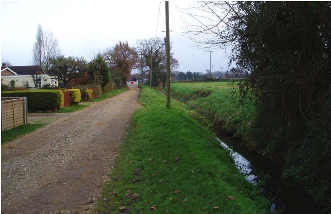
Figure A.11: Flowers Lane Drain Looking Downstream Towards the Railway
