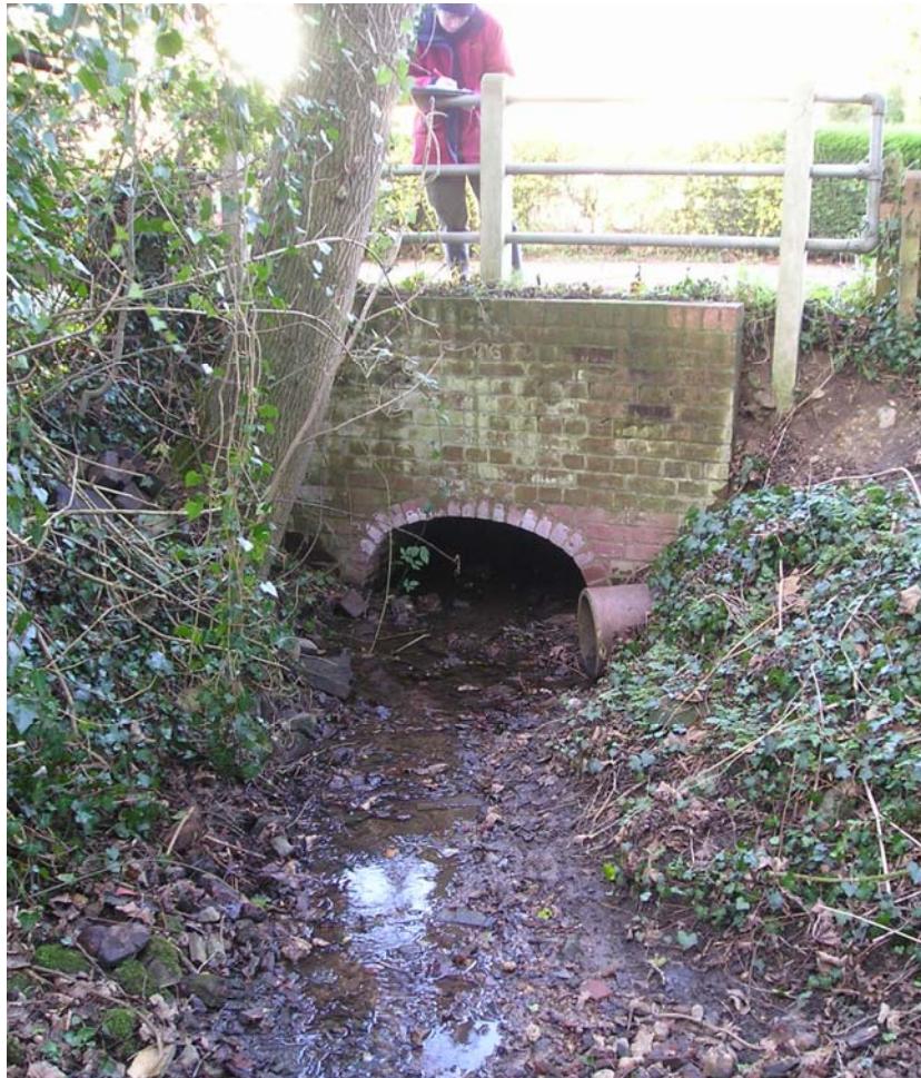
Figure B.5: Moat Stream looking downstream to Dereham Road Bridge
