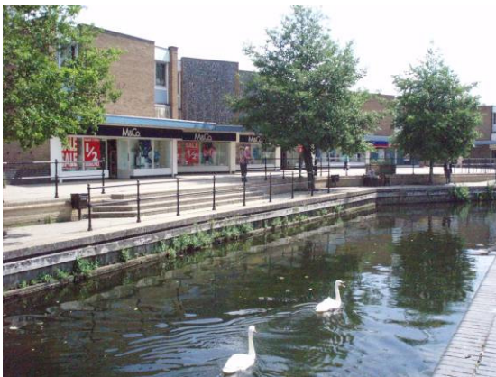
Photo 7: Standing on left bank looking towards existing shopping precinct. Two stage channel is again apparent. Man-made river bank consists of timber structure with concrete crest.
