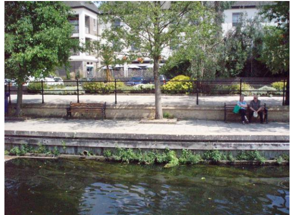
Photo 6: Standing on the left bank looking across the river. Two stage channel is apparent along the riverside providing pedestrian access. Private car park and hotel is located beyond.
