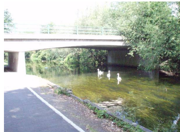
Photo 4: Standing on left bank, looking downstream towards the A1075 Road Bridge. Supermarket car park located on right bank upstream of road bridge.
