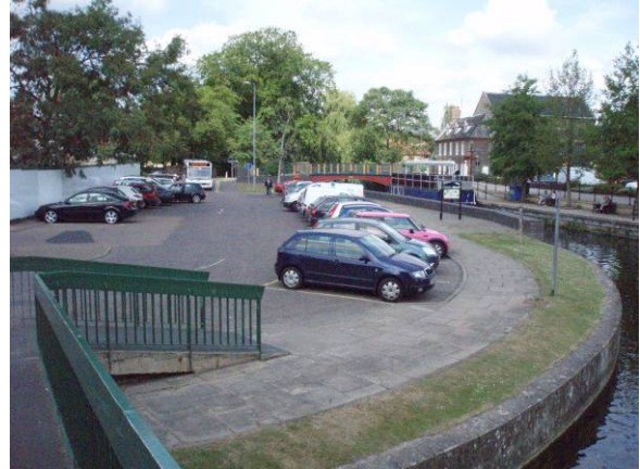
Photo 18: Standing on foot bridge, looking north west towards existing car park. Man-made concrete wall exists along the river bank (raised in sections).
