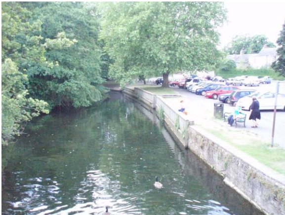
Photo 19: Standing on foot bridge, looking upstream of river. Man-made masonry wall with raised concrete wall sections exist along the river bank.
