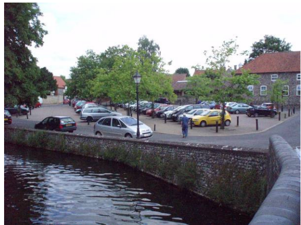
Photo 14: Standing on bridge along Bridges Walk, looking downstream towards area of interest 3.
