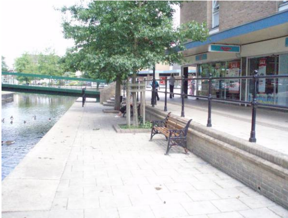
Photo 9: Standing on right bank, looking north towards foot bridge, with shopping precinct on right. The two stage channel continues in this location, providing pedestrian access along the riverside.
