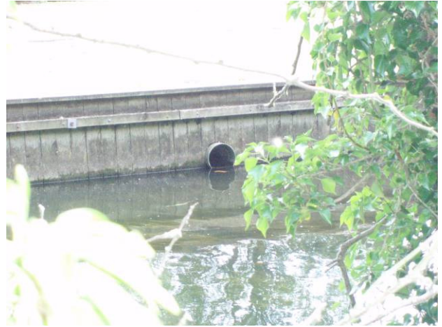
Photo 10: A number of surface water outfall pipes are situated along the riverside within this area of interest.
