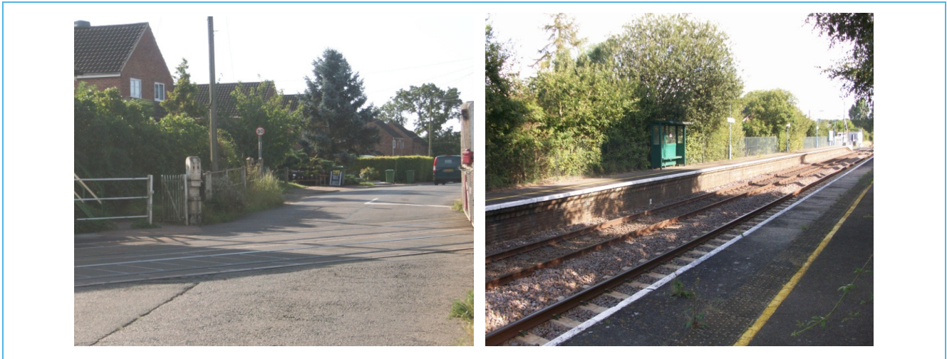
Figure 13 Lack of provision for pedestrians over the level crossing (left) and existing platform shelter (right).
