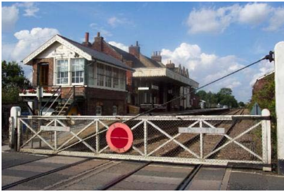
Figure 4.7 – Attleborough Rail Station
