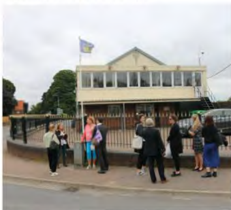
1.6 Queen's Hall, a valuable community asset, is surrounded by railings and a lack of active ground floor frontage which hinders a positive relationship with the street
