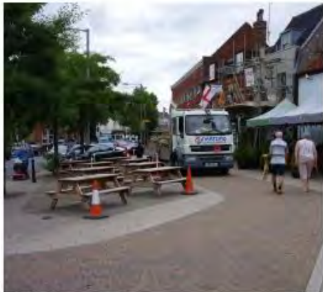
2.1 Newly paved shared surface is not legible and thus contested by pedestrians and vehicles
