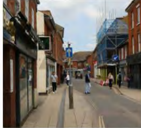
1.3 The town centre would benefit from public realm improvements - restricted pavement widths, cluttered walkways and ineffective drainage solutions impact on pedestrian movement
