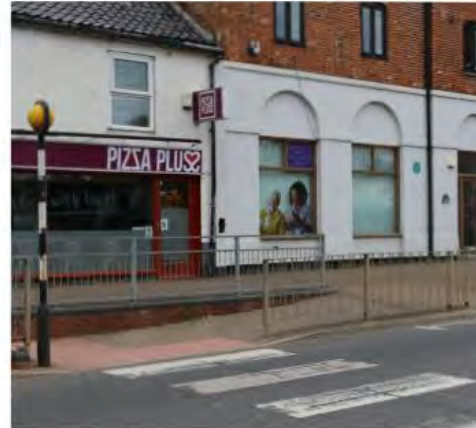
1.3 One of two zebra crossings on Watton High Street has an uneven camber that makes crossing precarious for those in mobility scooters and wheelchairs
