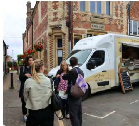
1.7 Town Hall and museum is a listed building, but could be improved by rethinking how it addresses the market and public realm. The entrance is currently hidden
