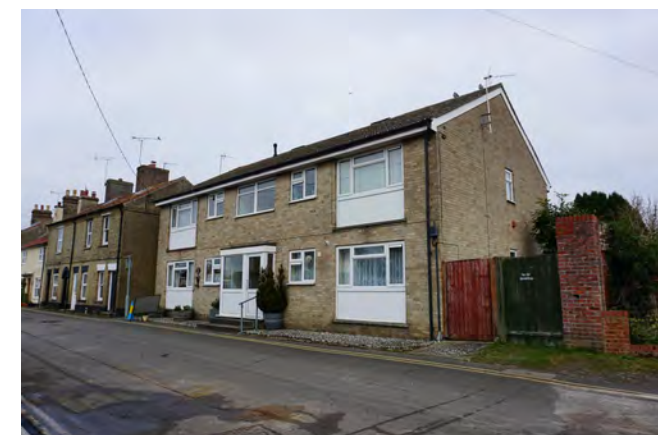
Modern house to be removed from the boundary
