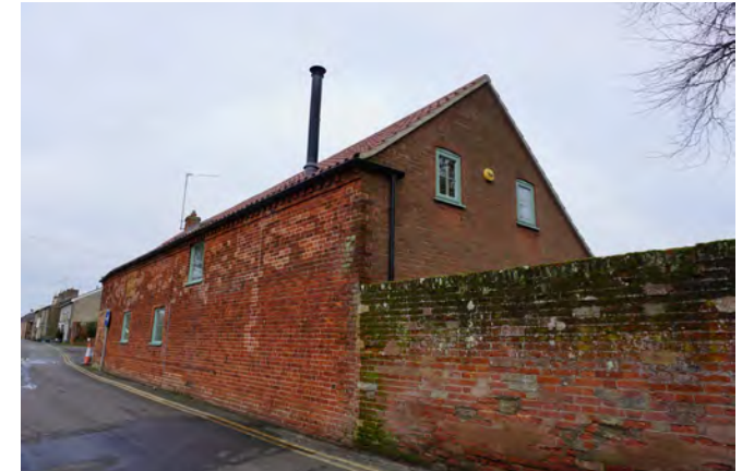
Converted outbuilding to be included within the boundary
