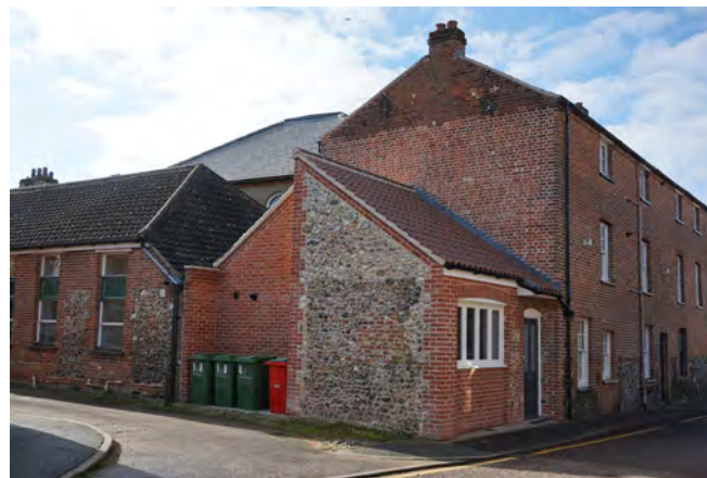
Built-in bin storage area in new extension on Pit Lane
