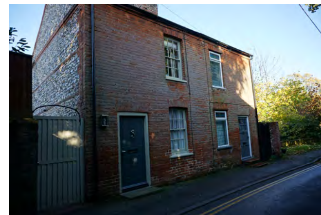
Nos.1 and 3 Northwell Pool Road
