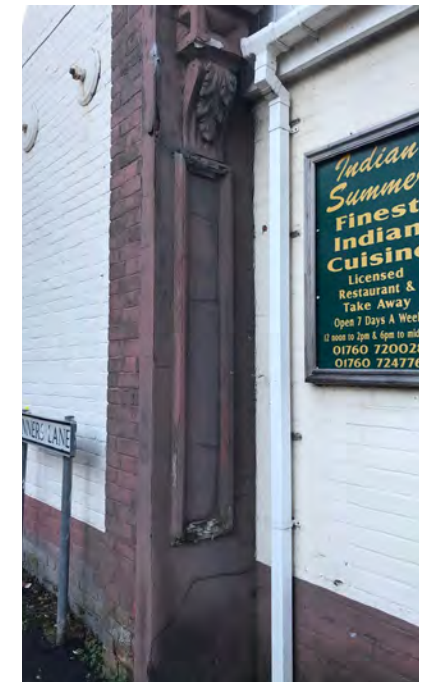
Pilaster of the historic shopfront on Station Street which still remains
