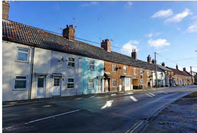
A View along terraces on Lynn Street
