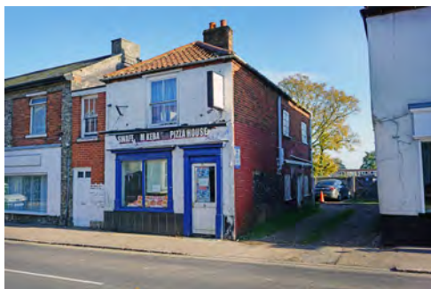
Poor quality signage and windows stickers, though the historic shopfront is good quality and could be revived with better maintenance and signage
