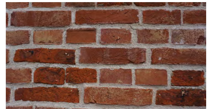
Good quality re-pointing using lime mortar
