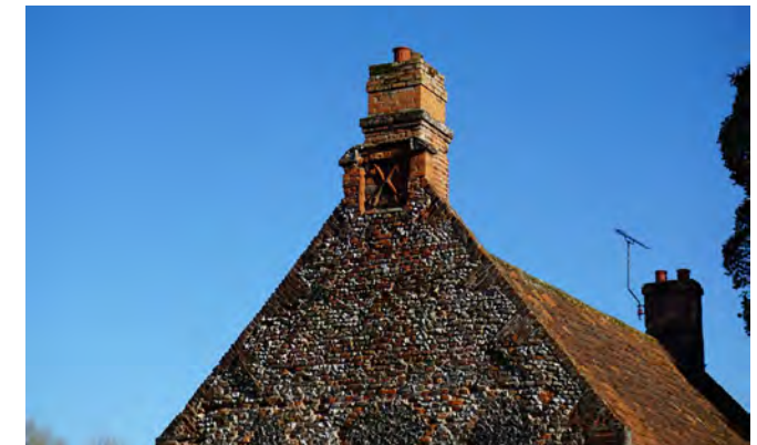
An example of a building on Mangate Street using flint with red brick pattering on the gable end, with a red brick chimney and red clay pantiles to the roof
