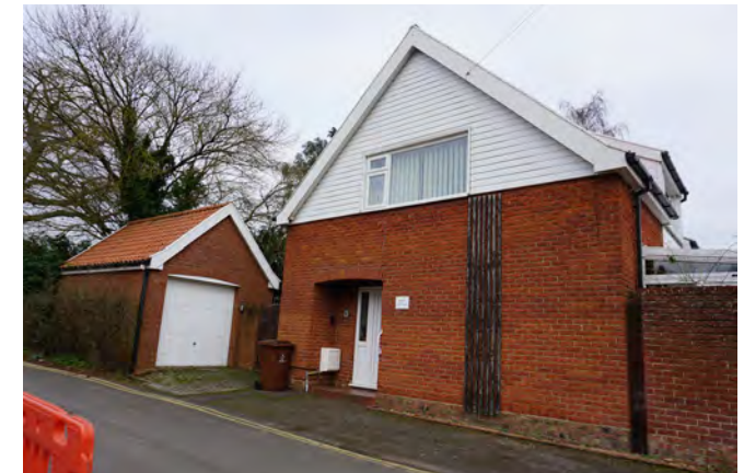
Modern house to be removed from the boundary
