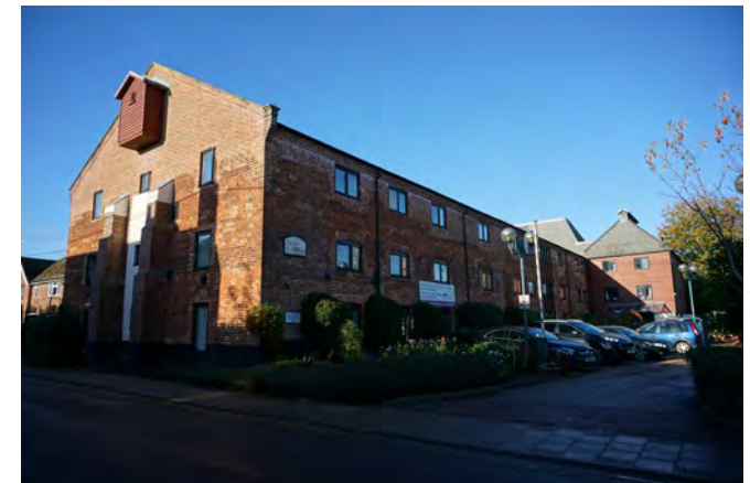
The converted Maltings
