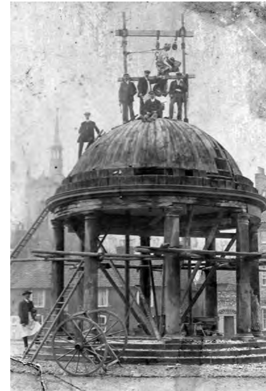
Restoration Work of Butter Cross c.1910 (courtesy of Swaffham Heritage)
