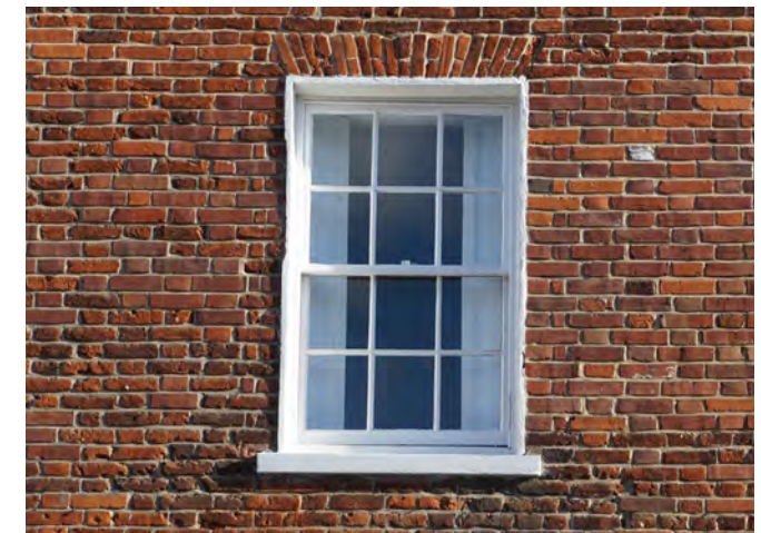
An example of a well-maintained historic timber sash window
