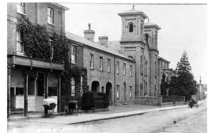
The Baptist Church in the late-nineteenth/early-twentieth century, also showing Nos.30-36 and No.40 Station Street (Courtesy of Swaffham Heritage)
