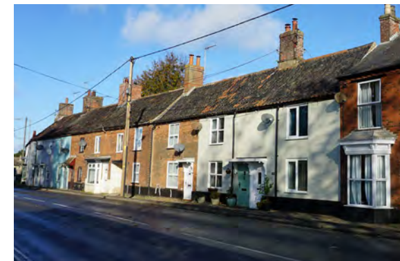
Multiple satellite dishes create a cluttered appearance
