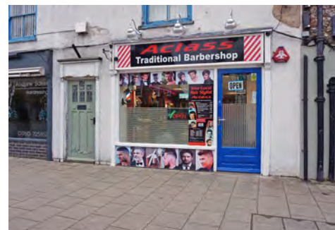
Garish plastic signage and multiple window stickers creating a cluttered appearance and blocking views into the shop
