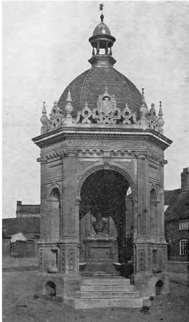
The Bagge Memorial c.1930s (courtesy of Swaffham Heritage)
