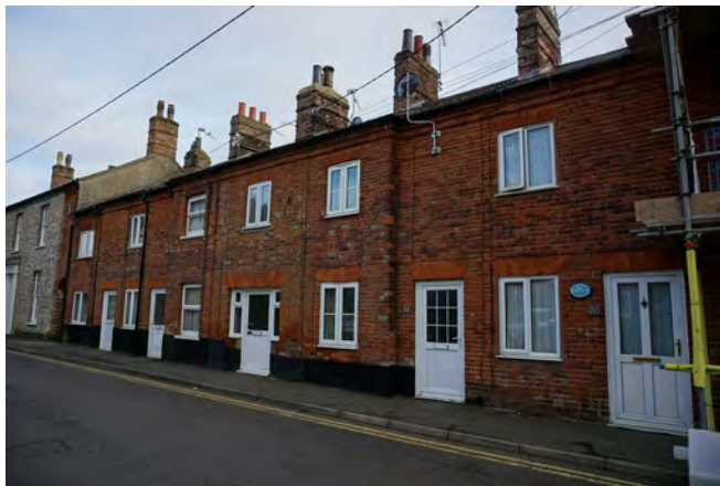
Terraced housing on Cley Road
