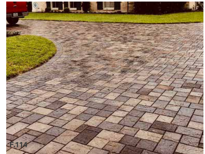
Figure 114: A good example of permeable paver (Source: https://www.paverconnection.com/testimonial/hedwig-village-permeable-driveway-and-patio-upgrade/ )
