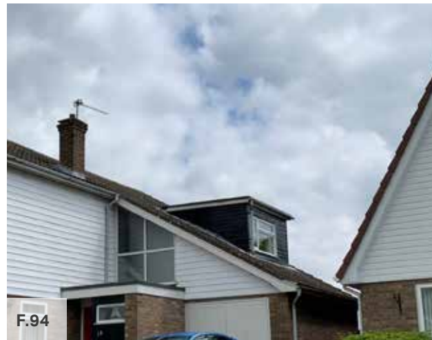
Figure 94: Ill-placed and out of proportion shed dormer
