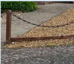
Gravel and concrete
