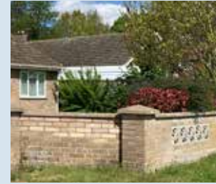
Gault brick wall
