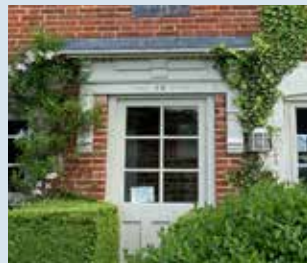
Flat roof porch feature
