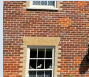
Sash window with lintel above
