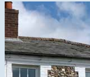
Slate tile roof
