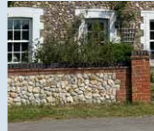
Flint and red brick wall with shrubs
