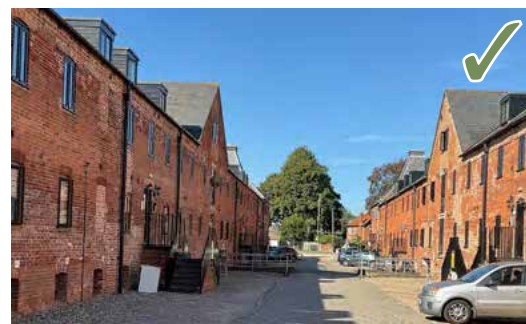
Existing buildings of heritage value that contribute to local character, converted from industrial to housing. Dereham Maltings conversion.
