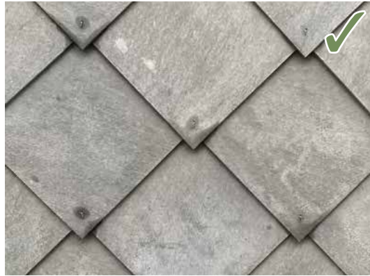
Materials should be durable, lightweight and reclaimed where possible e.g., fibre cement tiles
