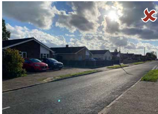
Wide, straight roads with few defining features often encourage vehicles to speed, and should be designed out of new development as seen in this example in Attleborough.
