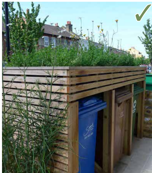
Bin storage is integrated into the front garden, easily accessible, and screened from the street view.
