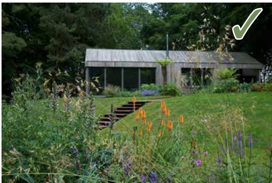
A simple building form is employed in this eco home, which reflects a traditional barn typology © Photo Ricard Hanson for Jeremy Stacey Architects
