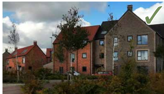
Well-proportioned, gabled building with a contemporary pattern of openings that are generous, relate to the interior and create a rhythm of openings on the façade, Norwich
