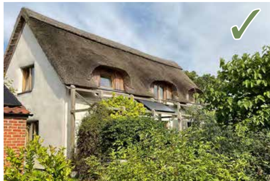
A simple building form that is a contemporary interpretation of a traditional timber frame house. Dormers add complexity but contribute to local character. This is an example of a Passivhaus. Hickling © Fran Bradshaw of Anne Thorne Architects
