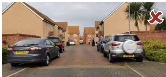
Parking should be designed so that it does not dominate the street and footways.
