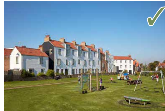
A terrace of taller buildings define and overlook an existing town green in Suffolk (© Ash Sakula).
