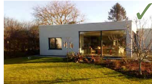
Passivhaus principles should be combined with innovative design quality to reduce overall energy consumption in new development - Yaxham.
