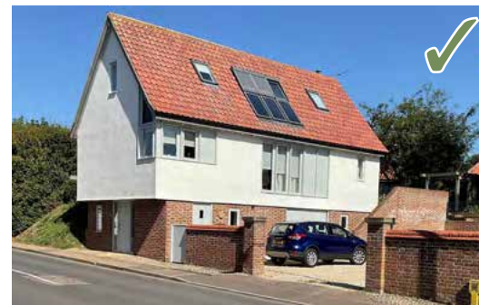
Contemporary interpretation of timber framed housing with simple compact form, articulated only by a jettied first floor. Wymondham © Lucas Hickman and Smith
