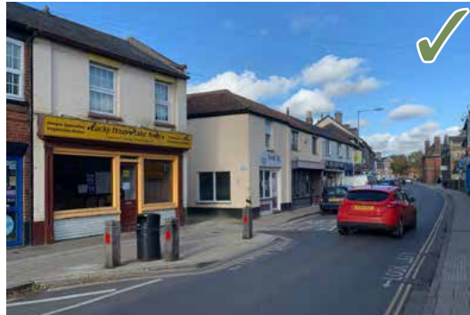
Carriageway narrowing example, Attleborough.
