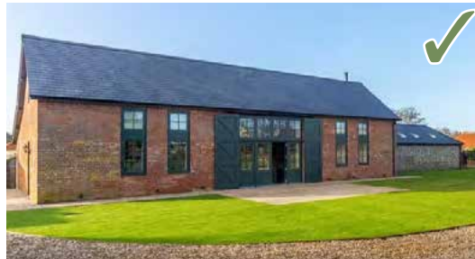
A contemporary interpretation, retaining the scale of the historic barn door opening with large windows, dark coloured mullions and transoms and large timber doors, Norfolk.
