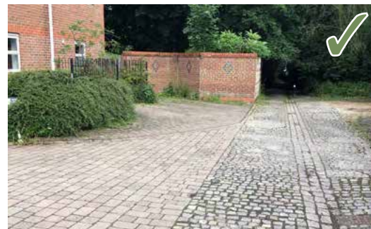
Re-used or re-claimed setts add richness to the character of the street in a new development. Norwich
