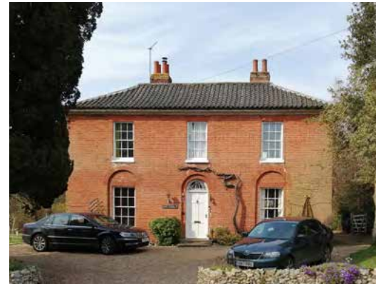
Well proportioned Regency villa with generous floor to floor heights, a shallow roof with projecting eaves, a hierarchy - elegant and varied window proportions, depth created by arched surrounds, reveals and timber sashes, and an attractive red brick.
