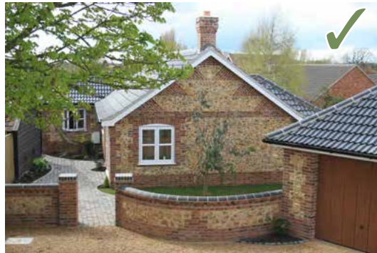
Texture, detailing, and materials have been used to create characterful façades in this example in Shipdham. © Clayland Estates
