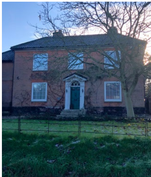
The Madingley, Dereham Road, a Grade II listed residential building. The architectural materials and features, particularly the red Norfolk brick, clay pantiles, and white fenestration, are typical of Mattishall.
