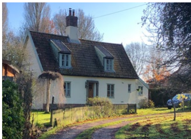
Traditional style house on Church Lane, Mattishall Burgh. The cream render, vertically proportioned dormer and sash windows, tiled roof and narrow brick chimney are locally distinctive. The building is well set back from the road on a large plot.
