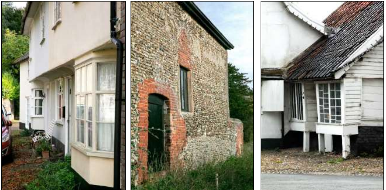
Figure 9 Some of New Buckenham's historic buildings
