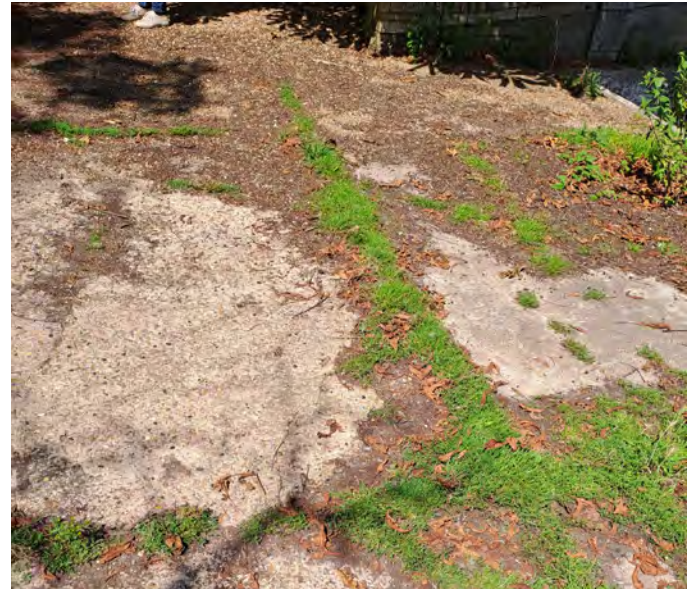
Cracked and uneven concrete slab by the river at the east boundary of the Conservation Area
