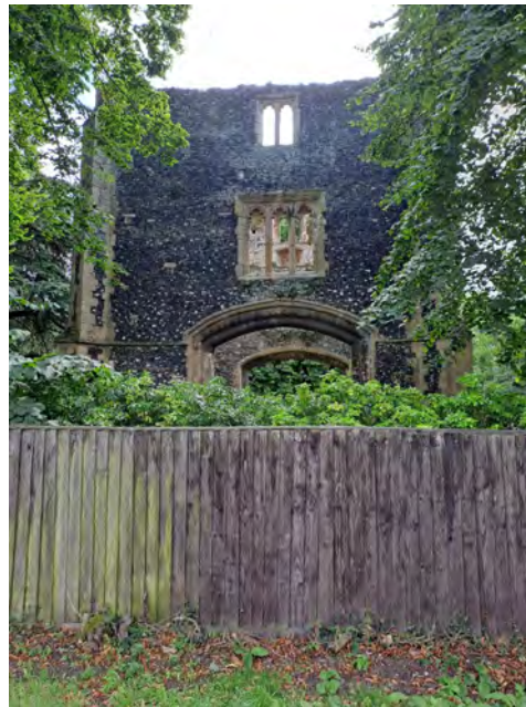
B Glimpsed view of the Priory Gatehouse from Abbeygate
