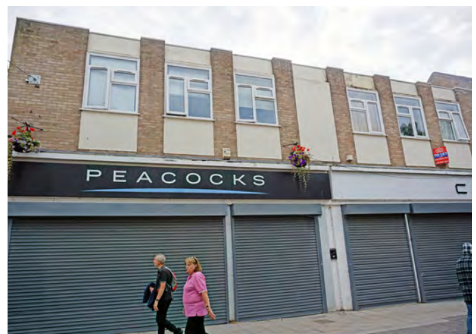
Long façade across several historic building plots with roller shutters unsympathetic to the Conservation Area
