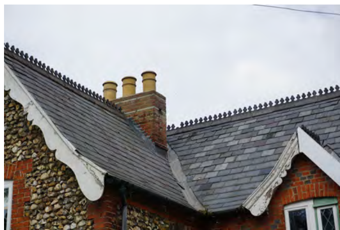
Historic bargeboards and ridge tiles on Old Market Street
