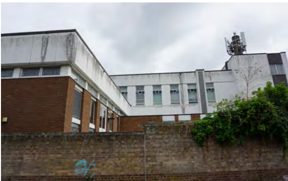
Large telephone exchange out of character in scale and style
