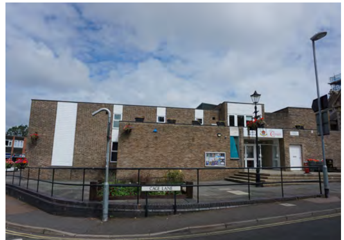
Poor landscaping around the Carnegie
