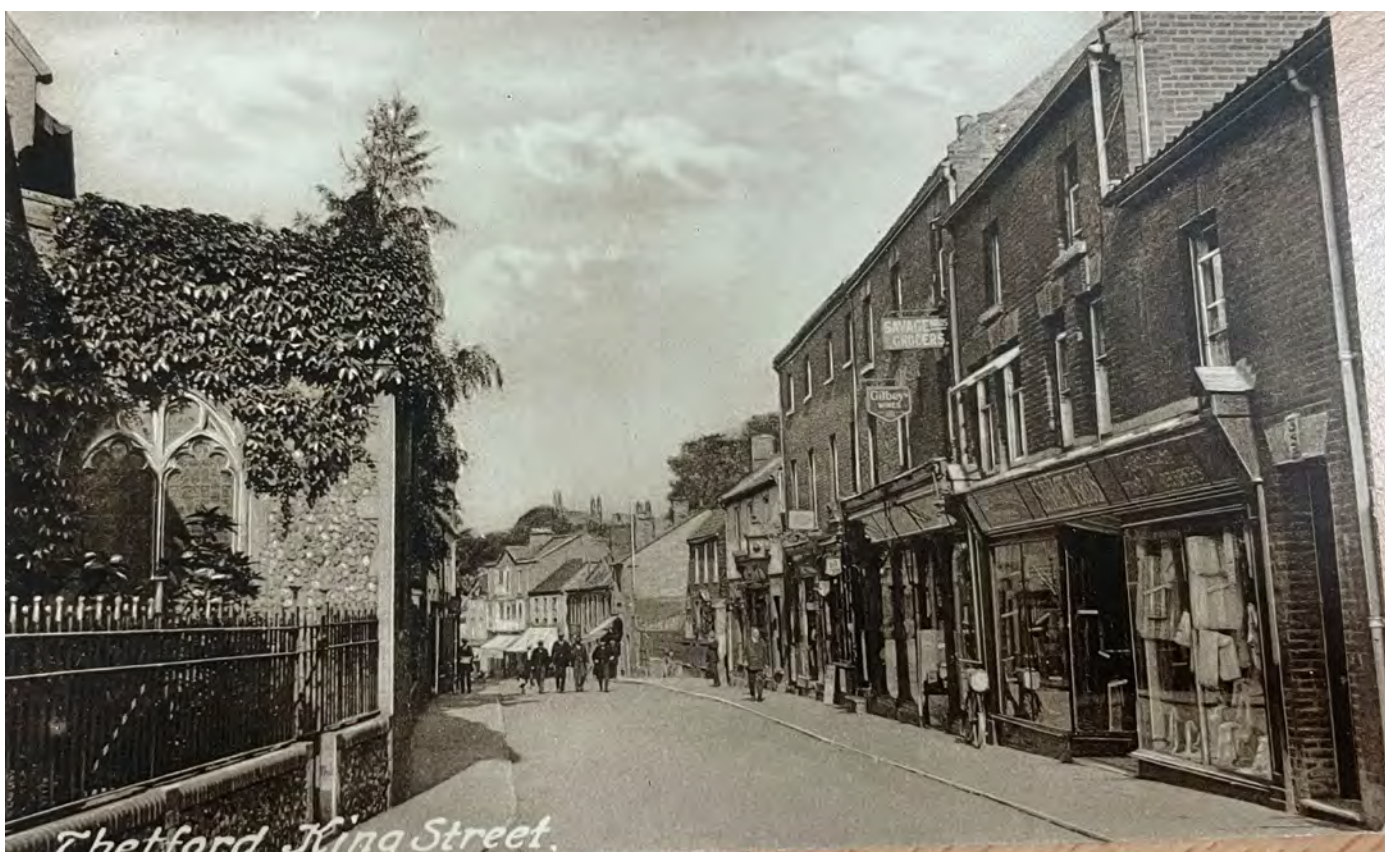
Shops on King Street, early twentieth century (Ancient House Museum)
