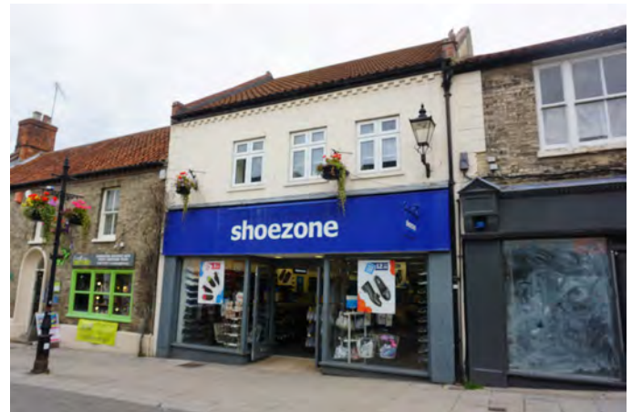
Overly large fascia with large stickers creating a cluttered appearance
