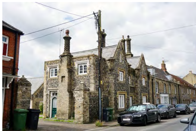
Decorative chimneys on Ford Street
