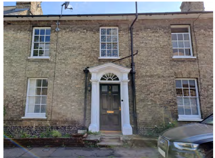
Medium Sized house on Old Bury Road
