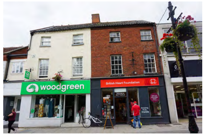
Garish signage out of proportion to historic shopfront on the left. Large signs blocking windows on the right.
