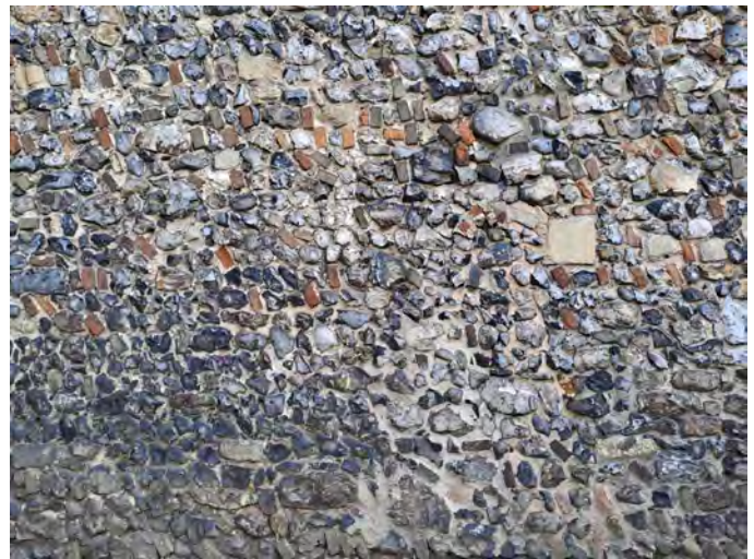
Monastic and ecclesiastic building stone incorporated into flint walls
