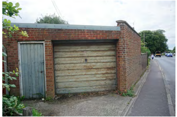
Roller shutter garage door on Bury Road
