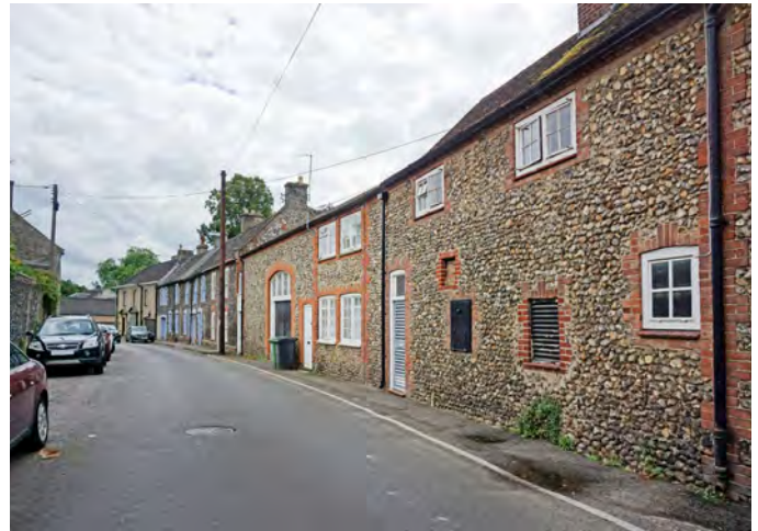
Lack of paving around Ford Street
