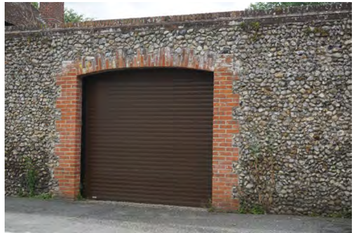
Roller shutter gate on Ford Street
