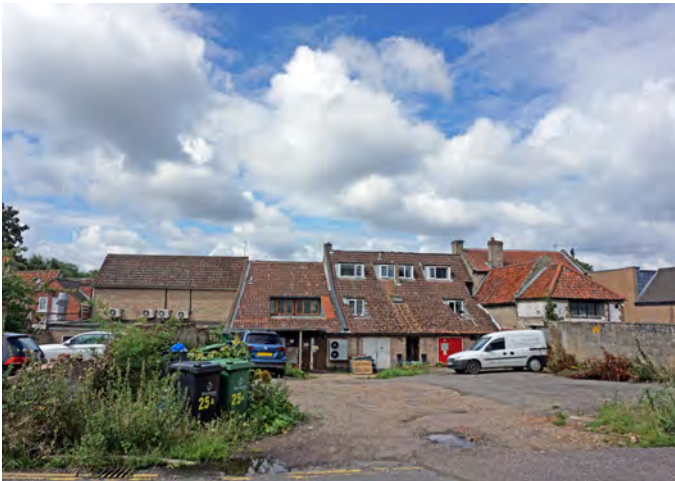
Run down areas to the rear of buildings fronting onto Guildhall Street
