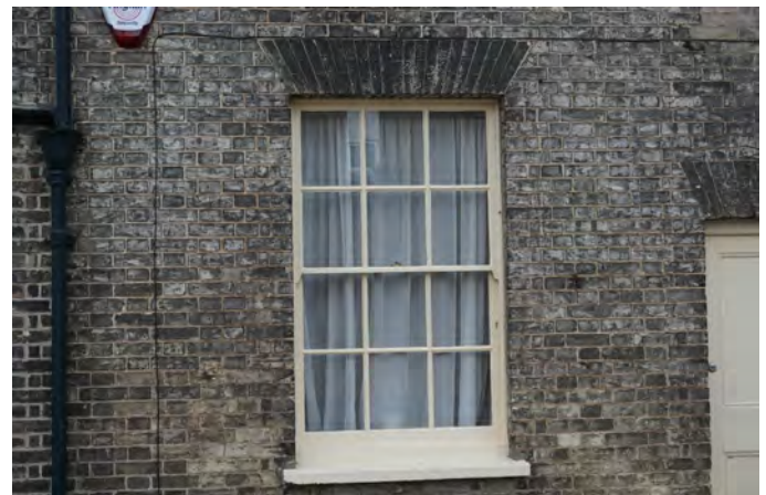
An example of a well-maintained historic timber sash window
