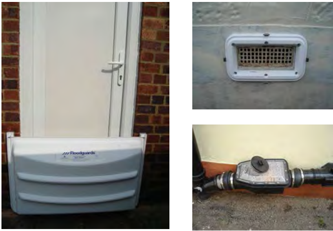
Figure 5-3 Examples of flood barriers, air bricks and non-return valves
