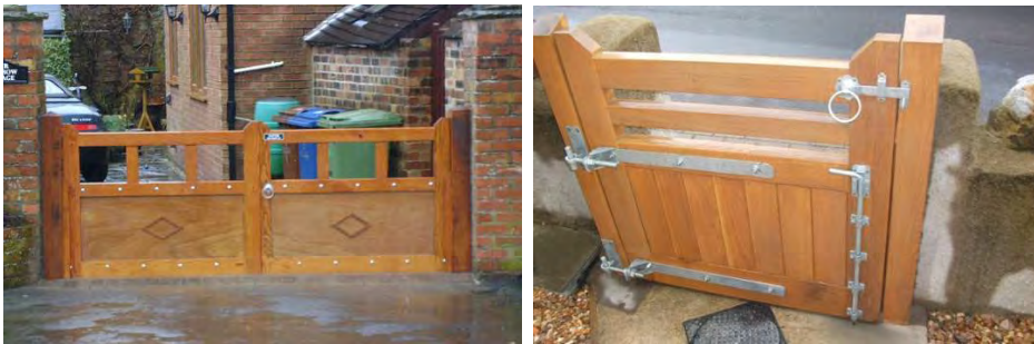
Figure 5-4 Example of flood gates
