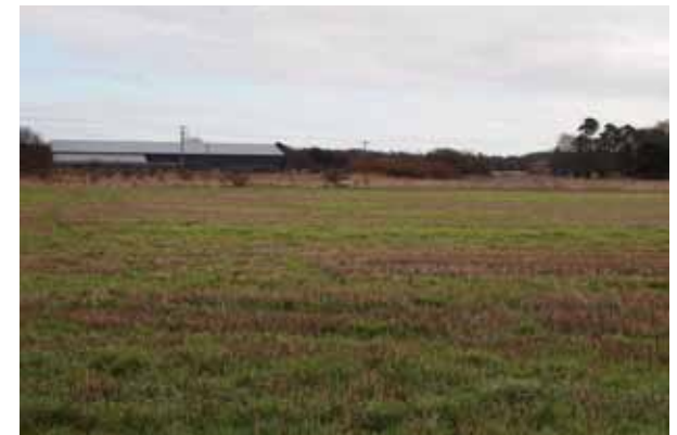
Large sheds and farm buildings can seem over scaled within the small-scale Settled Fen
