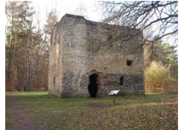
Thetford Warren Lodge was probably built around 1400 by the Prior of Thetford. It is a defensive building which housed guards who protected the rabbits of Thetford Warren from poachers.
