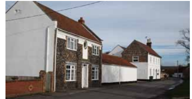
Traditional buildings in Hockwold - local materials are an attractive mix of brick, flint and white render
