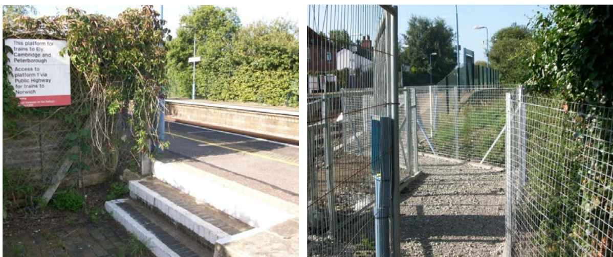
Figure 12 Access to Cambridge (left) and Norwich (right) Platforms.
