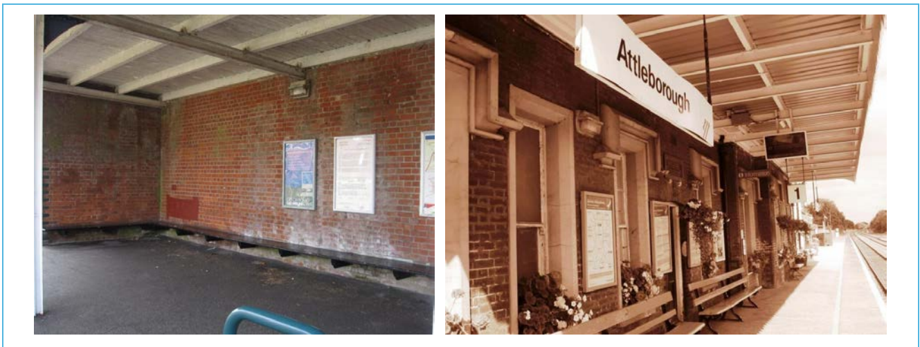
Figure 16 Shelter on Cambridge bound platform (left) and the canopy on the Norwich bound platform (right).
