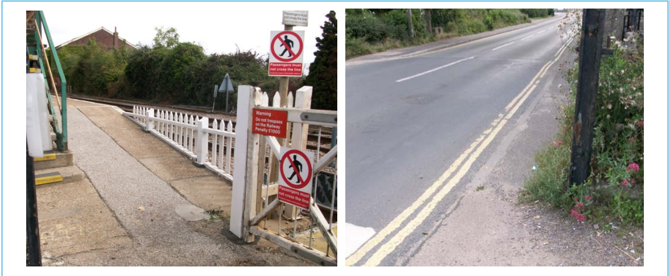
Figure 15 Entrance to Norwich Platform (left) and the footway entrance to Cambridge Platform (right).
