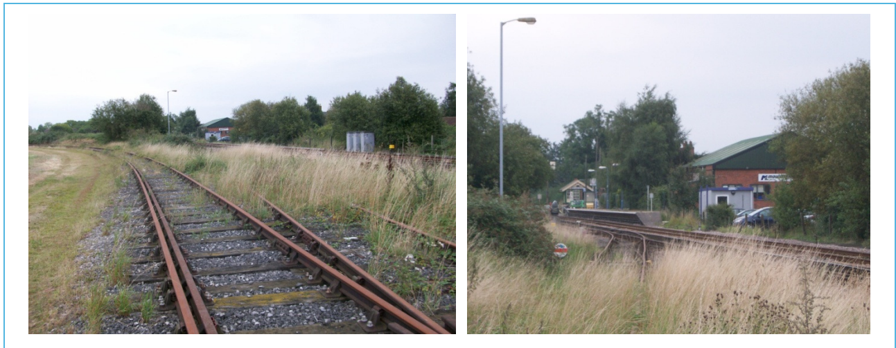
Figure 19 Private freight line (to the left in the photo) and main branch line (far right in the photo) (left) and connection with branch line at Eccles Road Station (right).
