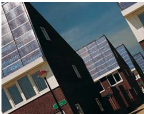
Urban design in the Nieuwland neighbourhood of Amersfoort, Holland, is centred on optimising solar potential
