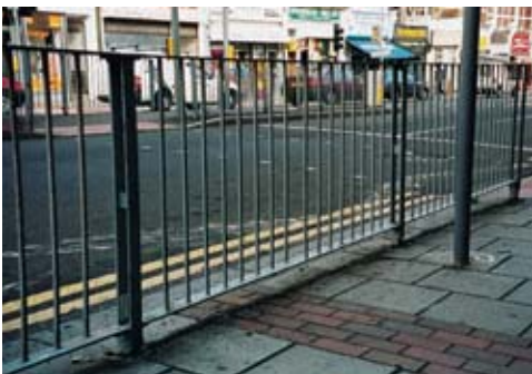
Sometimes facilities introduced in the name of 'pedestrian improvements' actually impede movement
