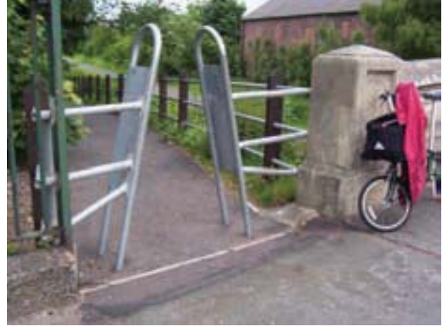
Figure 8.8 A-frame barrier (Steve Essex)
