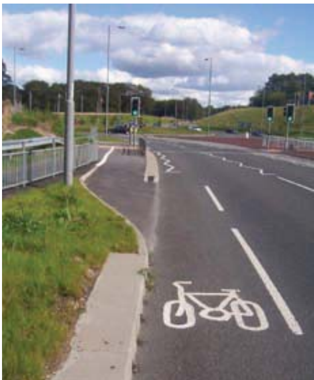
Figure 8.2 Smooth transition from carriageway to cycle track, Bingley. Note that the cycle symbol does not conform to diagram 1057 (see paragraph 3.3.2). (Tim Pheby)
