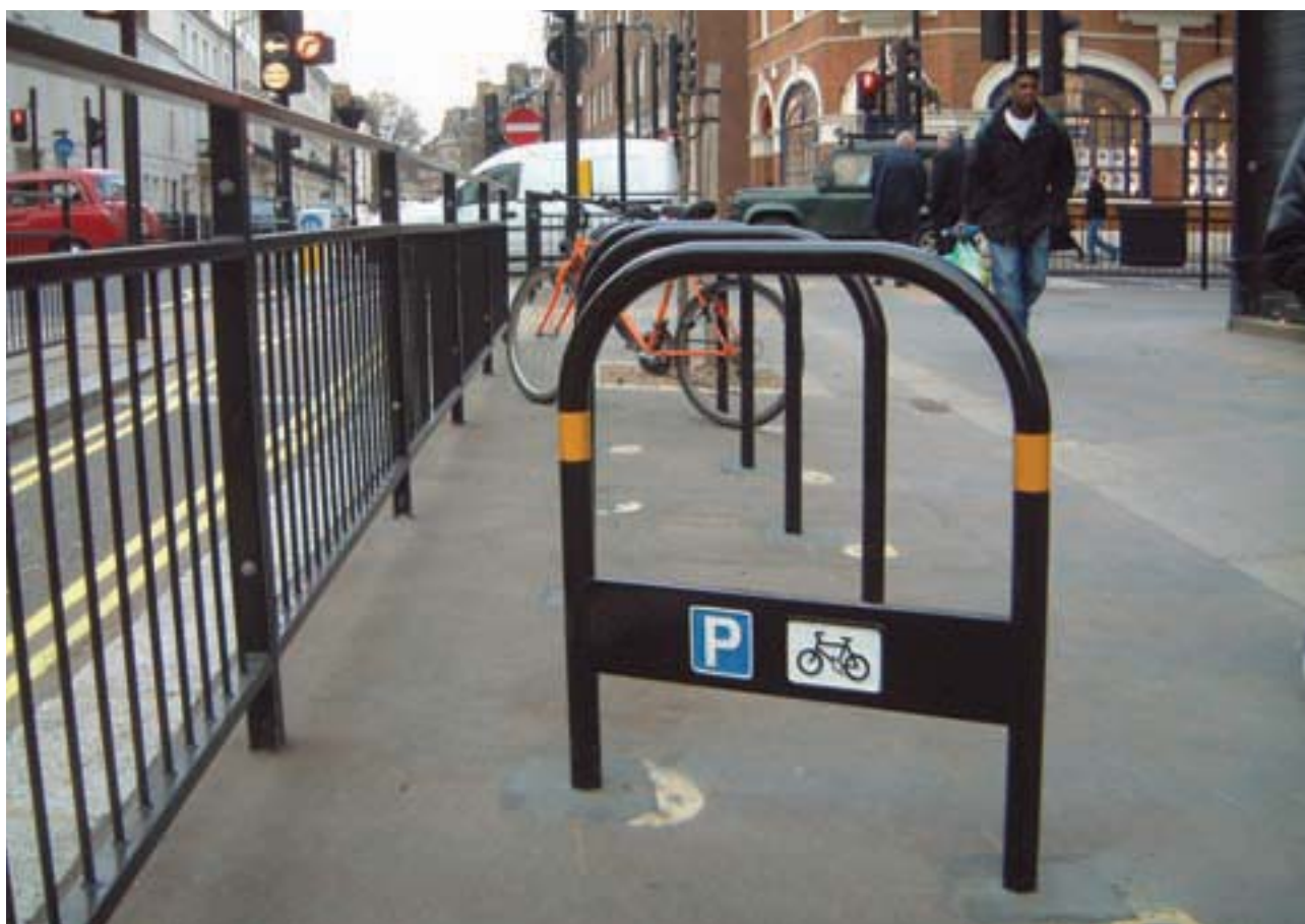
Figure 11.3 Sheffield stand with tapping rail and contrasting banding at beginning of row (Tony Russell CTC)
