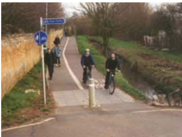
Figure 8.5 Bollard to prevent unauthorised car access (Alex Sully)
