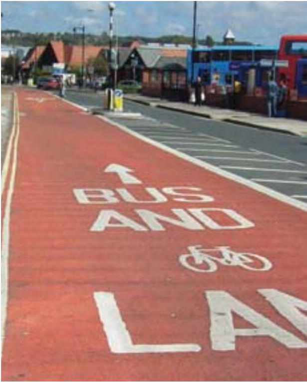
Figure 7.9 Contraflow bus lane, Isle of Wight (Patrick Lingwood)
