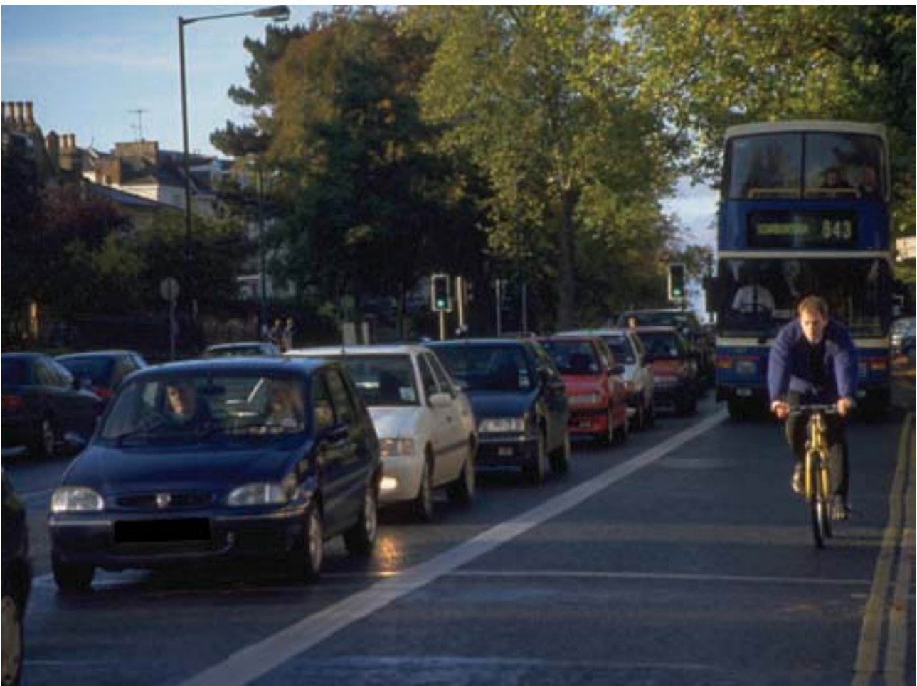
Figure 6.1 Narrow 3-metres wide bus lane (Sustrans)
