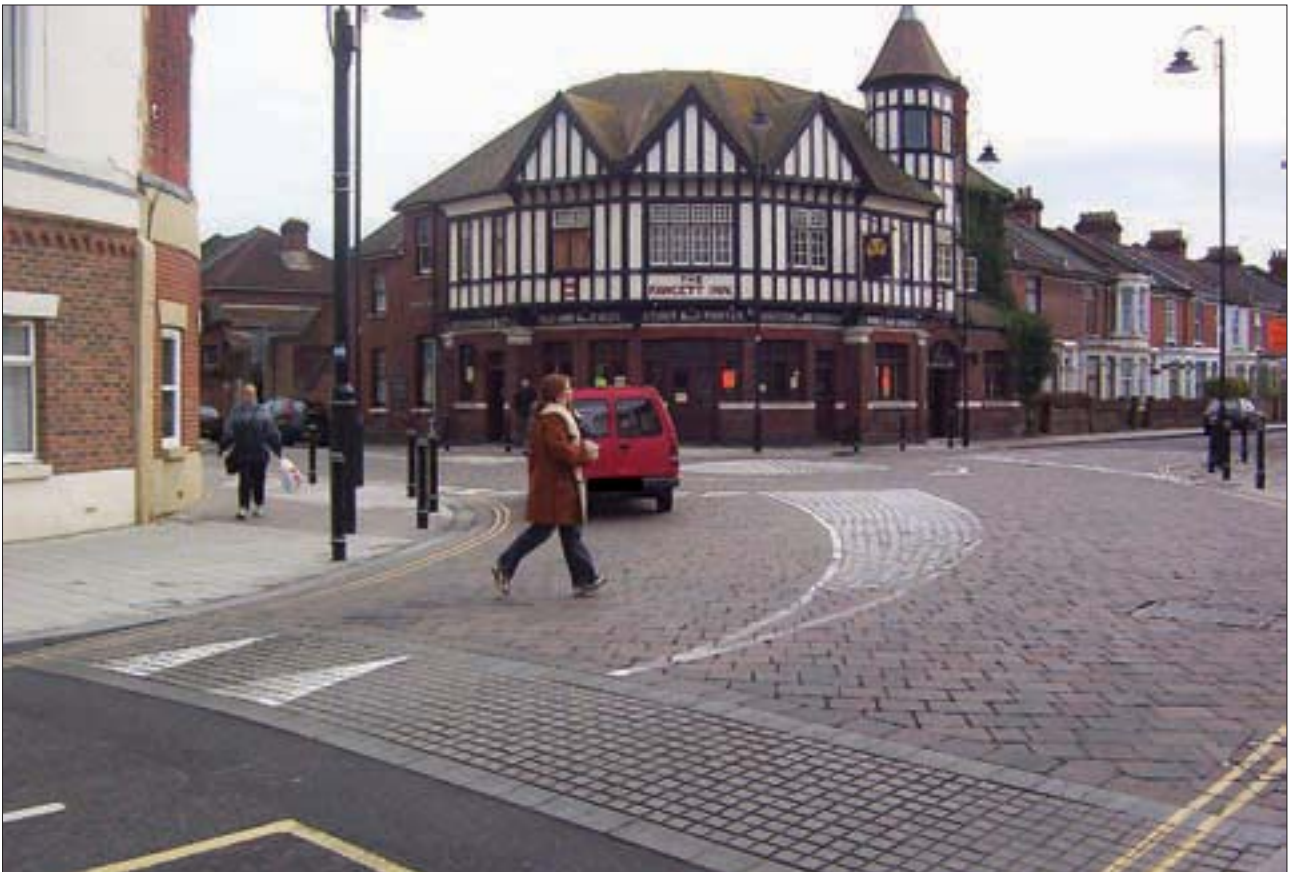
Figure 9.12 Mini-roundabout, raised junction and textured surfacing (Patrick Lingwood)
