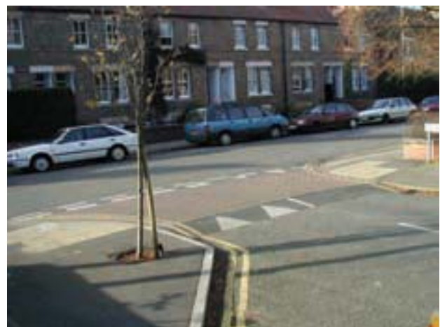
Figure 9.9 Localised narrowing and raised table at a side road junction (Patrick Lingwood)
