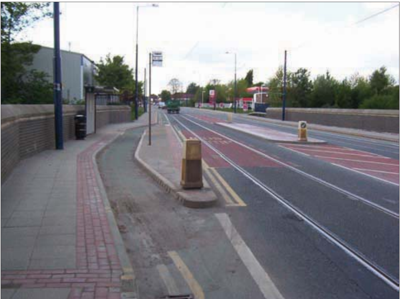
Figure 6.4 Cycle bypass at a bus and tram boarding island. The cycle bypass separates the bus shelter from the boarding area, and this may not be appropriate at busy stops where conflict with boarding and alighting passengers is more likely (Steve Essex)
