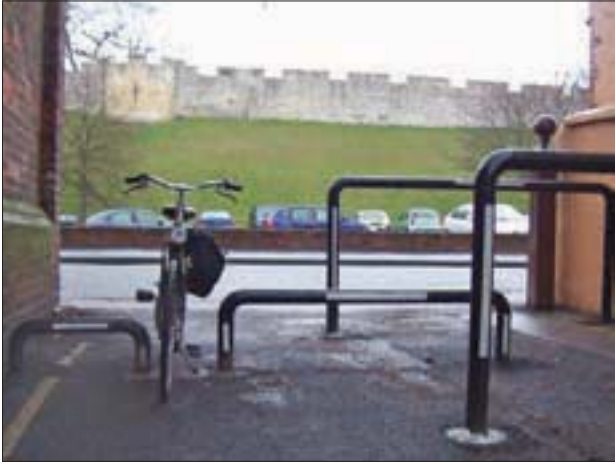
Figure 8.7 Barrier with wheelchair bypass (Tim Pheby)
