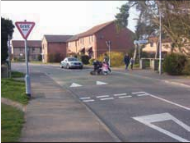
Figure 10.3 Cycle priority crossing over quiet road. Note that the sign to diagram 602 is incorrectly positioned (Rob Marshall)
