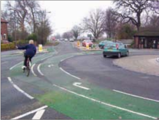
Figure 9.11 Roundabout with innovative cycle lane arrangement (Patrick Lingwood)
