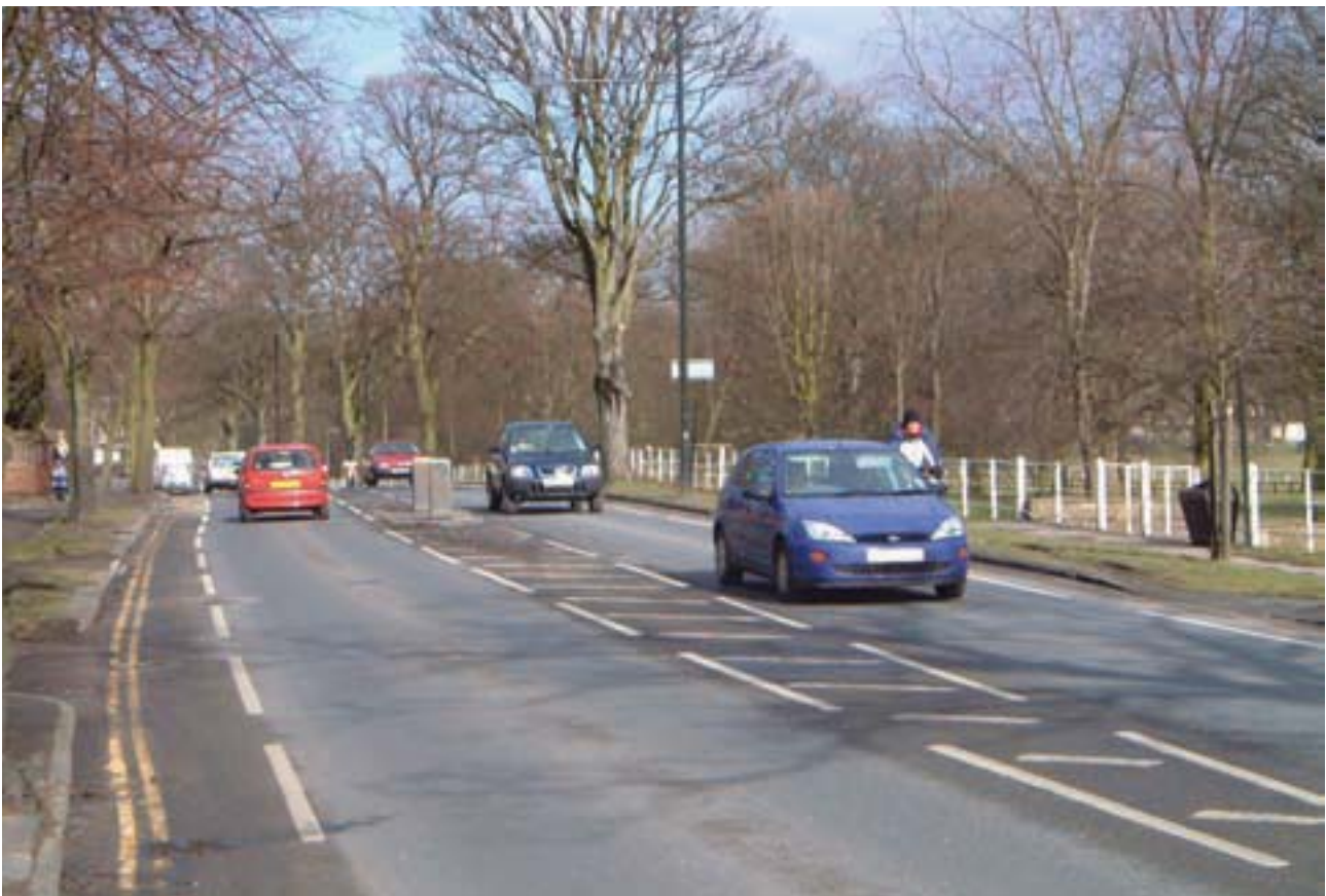
Figure 5.5 Cycle lane continued at refuge (CTC Benchmarking)
