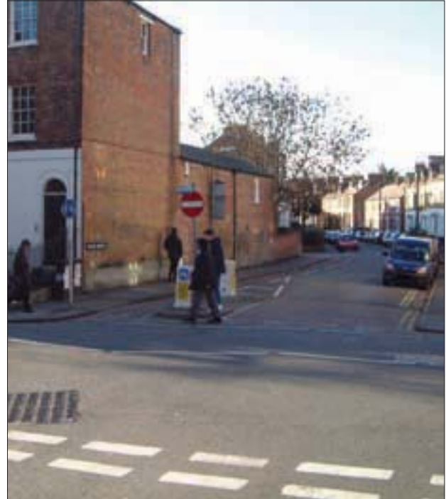
Figure 7.8 Refuge and segregated entry to cycle contraflow lane (Tony Russell CTC)
