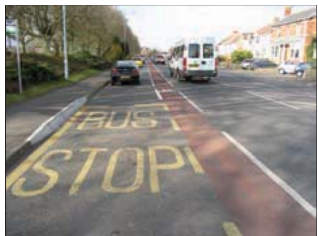
Figure 6.3 Cycle lane continued on the offside of bus stop and parking bays (Alex Sully)
