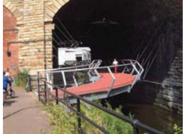
Figure 10.10 Cycle bridge suspended from a railway viaduct (Tim Pheby)
