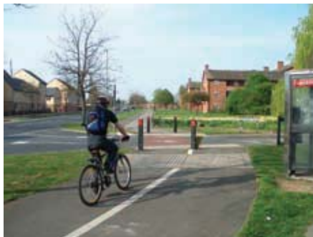
Figure 10.5 Bent-out cycle track crossing (Alex Sully)
