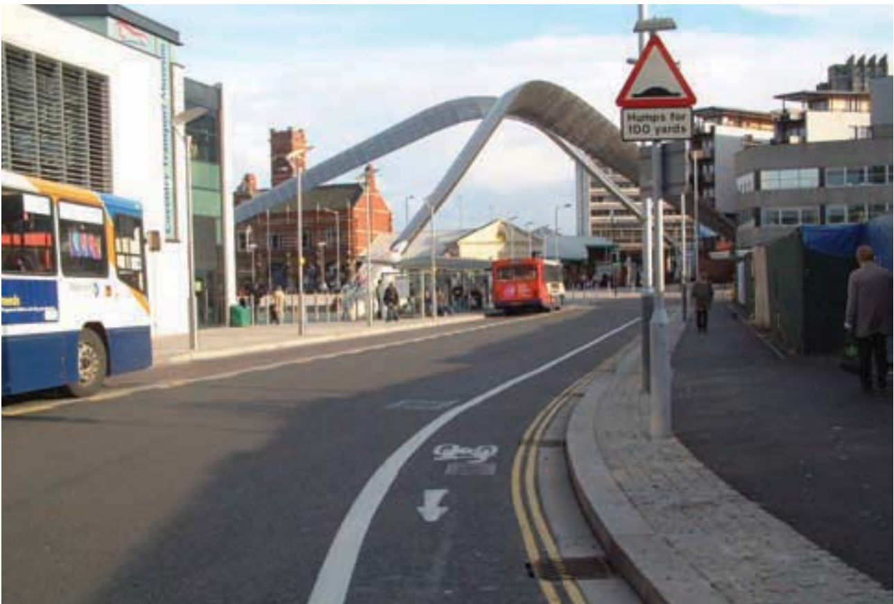
Figure 7.6 Mandatory contraflow cycle lane (Coventry City Council)
